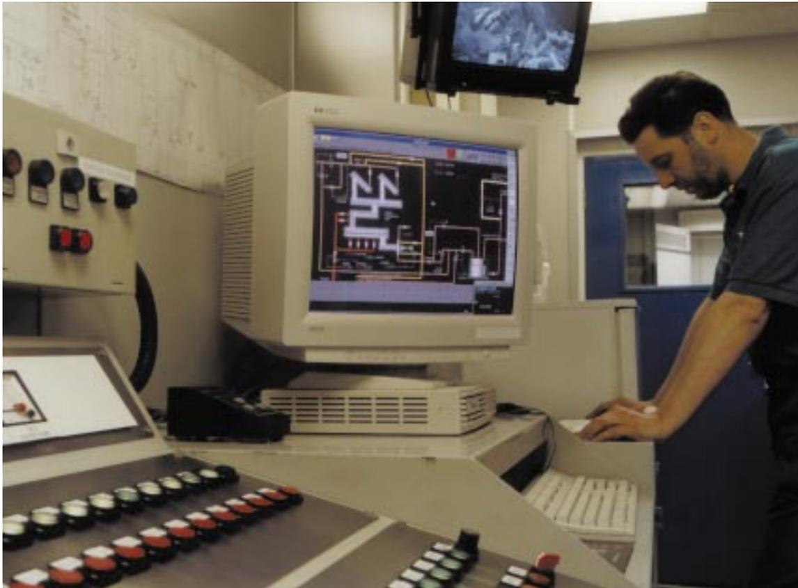
The AC 450 controller also interfaces to the existing S400 remote I/O in the stock preparation area simply by re-routing the Fieldbus.
