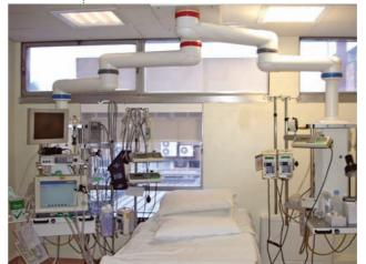
We also offer pendants specifically designed for the ITU/HDU, which include a docking system for connection of mobile ventilation anaesthetic trolleys to the service head if required. A full range of accessories for these pendants is also available to help make the most of your advanced pendants.
