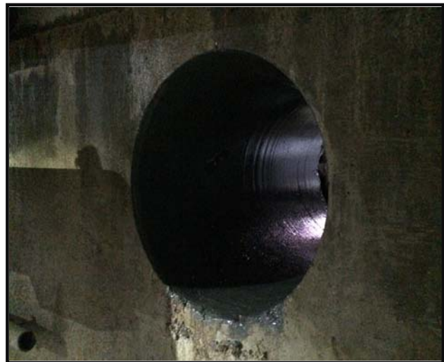
Fig 3 – New penetration through the detritor wall for the new odour control extraction duct
