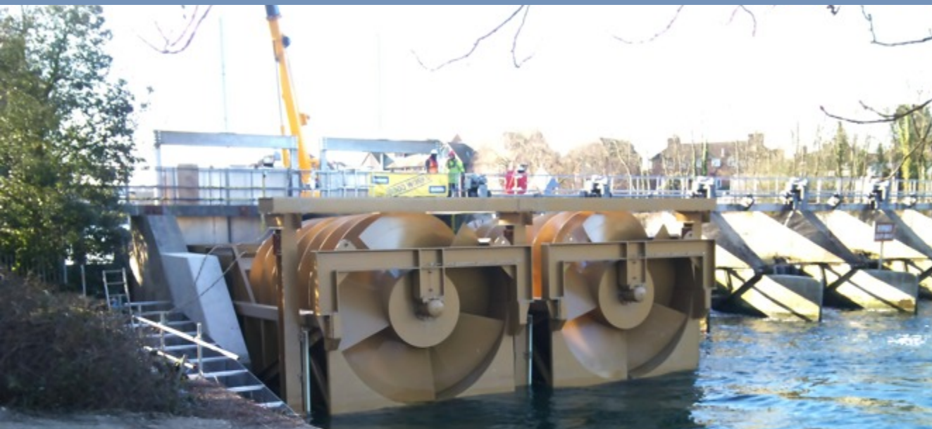
Also shown (right) is the new 3 stage screen Near Staines installed in January and below new stoplogs for the 30 year old failing weir at Iden Lock during design and structural analysis using our FEA software.
