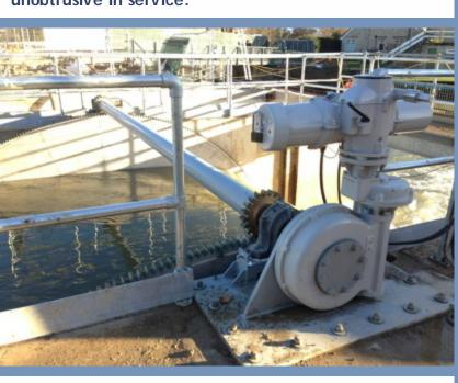
Adjacent to weir B above is the new weir A structure commissioned in December. This consists of 5 no handwound radial, supporting structure and pedestrian access gates over. The gates are shown the right in full service over the Christmas period.
