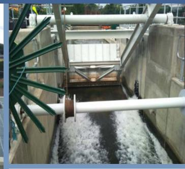
The summer period has remained a busy time for Huntons with continued works in river control and flood defence. Shown left and above we have the completed radial gate installation at Eldridges lock on the River Medway. The gate, designed and manufactured by ourselves is now complete and successfully controlling the upstream pen level to Tonbridge.
