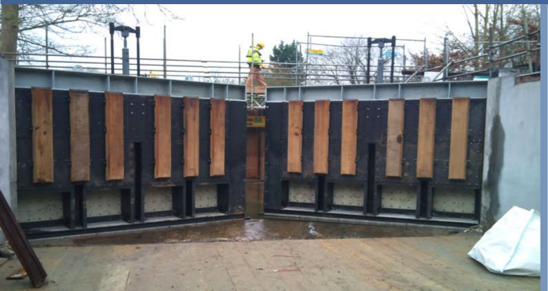
Our works on the Thames lock gate project has continued with the Manufacture and installation of new gates at Hurley lock. Shown left are the smaller head gates viewed from inside the lock. Shown below we have the fabricated blade of the new radial gate to be installed at Eledridges lock on the River Medway. Designed fully by ourselves the gate is now ready for installation next month.
